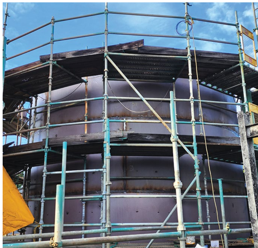
Water storage tank being repaired
