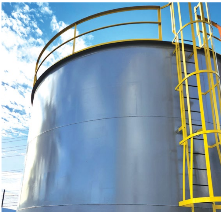
Repaired Fire Fighting Water Tank
