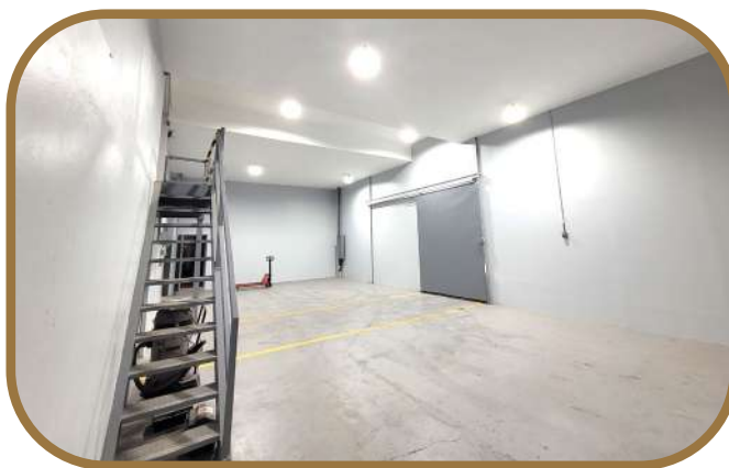
Inside of temporary warehouse
