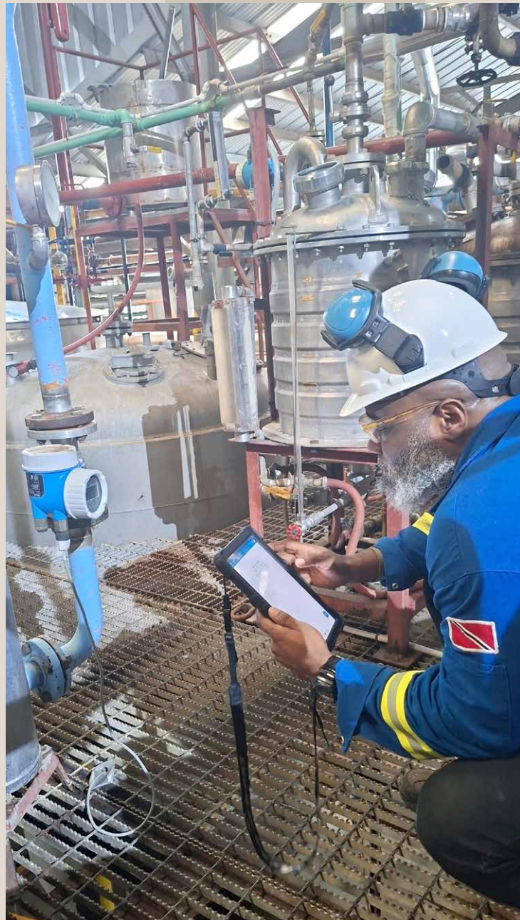
Distillery Operator completing digital operator rounds
